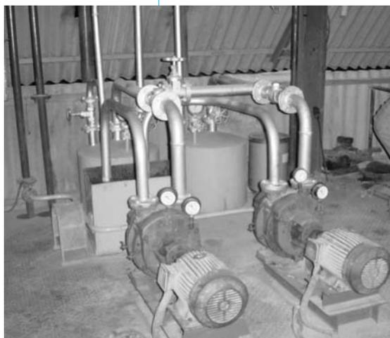
applications requiring rugged pump that can tolerate entrained liquids, vapors and fine solids. These Pumps operate in a liquid environment, generally water and are capable of handling vapors along with non-condensable loads.
