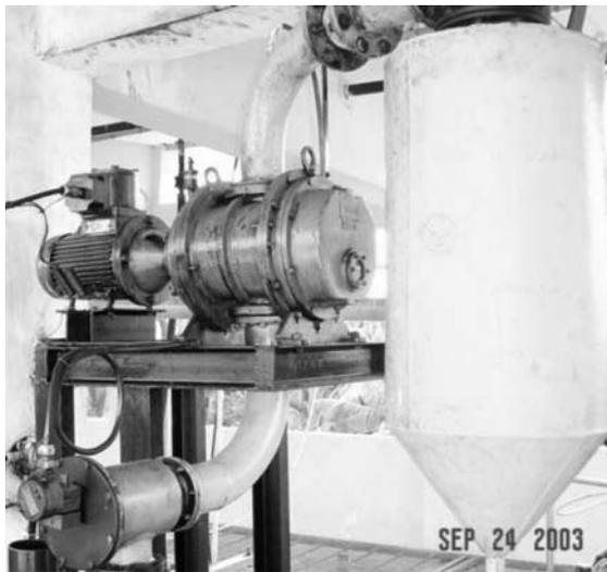
**DRY MECHANICAL BOOSTERS REPLACE STEAM EJECTOR**
