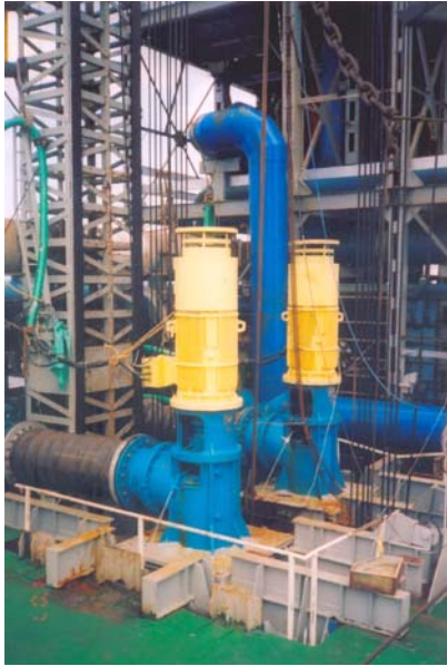
Fig 8 & 9: Cold Water Pumps of the Floating Barge Mounted Desalination System
