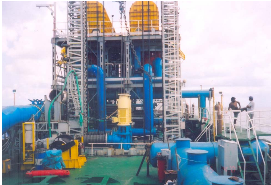
Fig 7: View of Floating Barge Monted Desalination System Aboard Sagar Shakti stationed near Chennai
