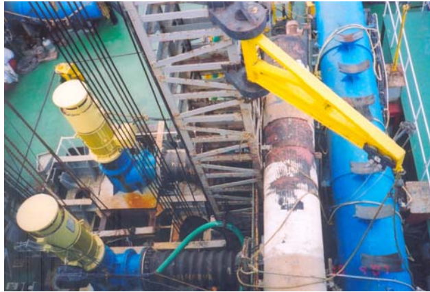
Fig 8 & 9: Cold Water Pumps of the Floating Barge Mounted Desalination System
