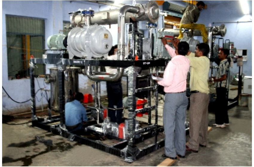
Fig 3: In-house F.A.T. (Factory Acceptance Test) being conducted to verify design parameters
