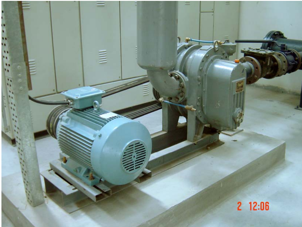
FIG: Typical Aeration Blower (Photo Courtesy: Everest Blowers, New Delhi, India)
