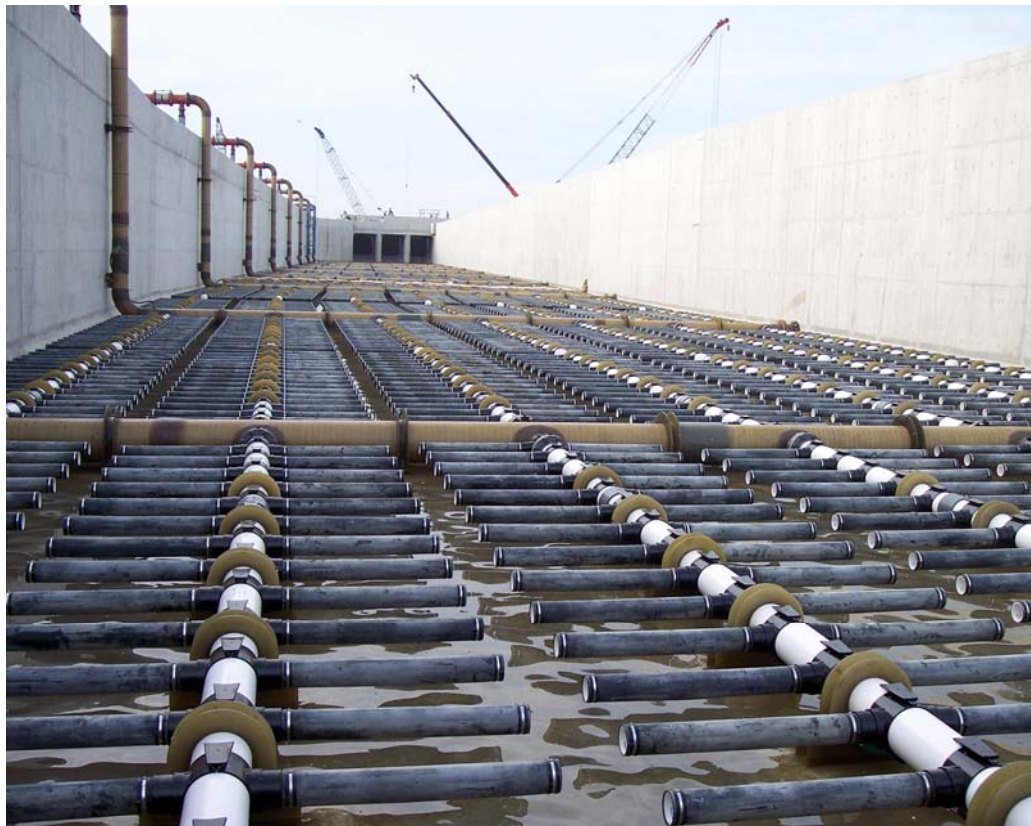
FIG: Tubular Diffuser Installation (Photo Courtesy: Environmental Dynamics, Inc., U.S.A.)
