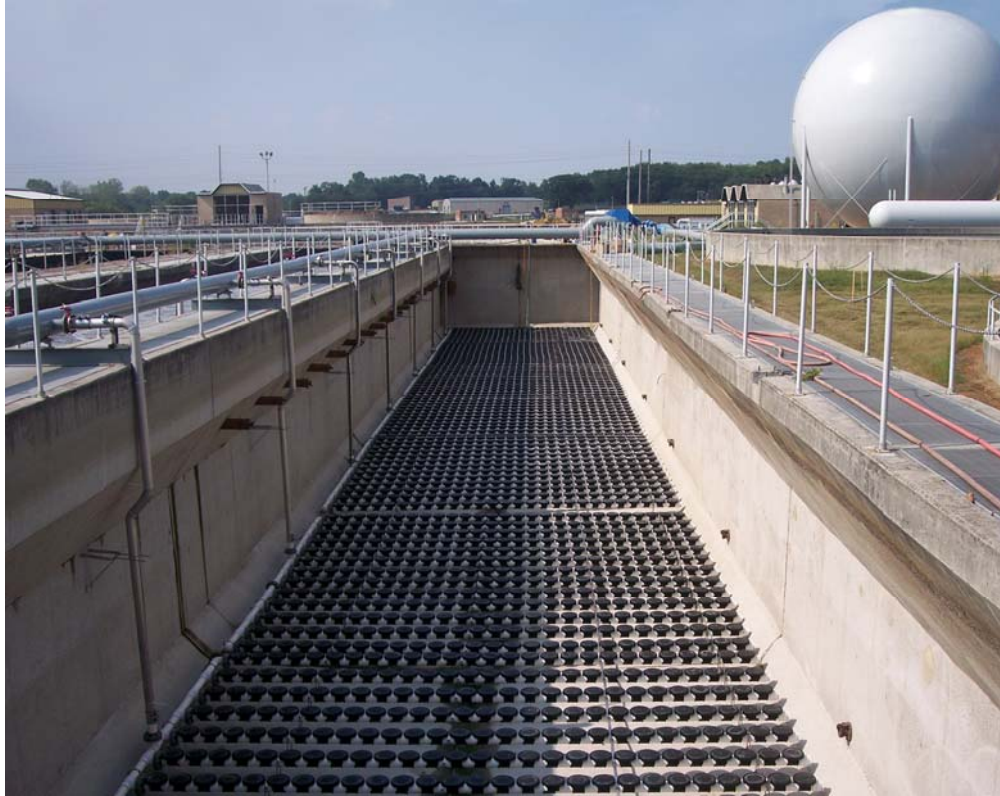
FIG: Disc Diffuser Installation (Photo Courtesy: Environmental Dynamics, Inc., U.S.A.)
