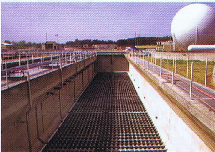
FIG: Disc Diffuser Installation (Photo Courtesy: Environmental Dynamics, Inc., U.S.A.)
